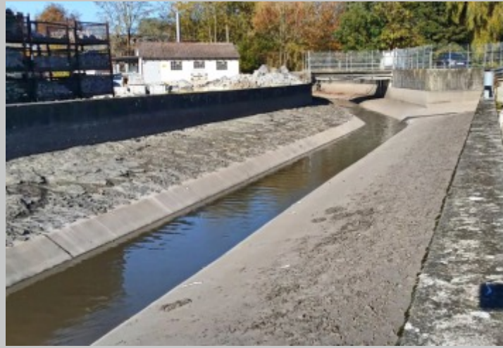
Situation on site
