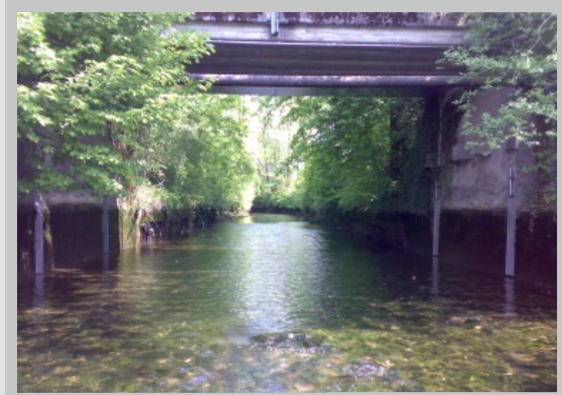
Measurement point at bridge
