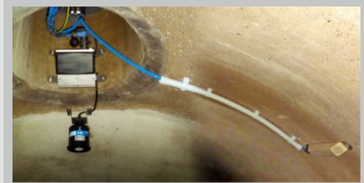
View of Measurement Place
