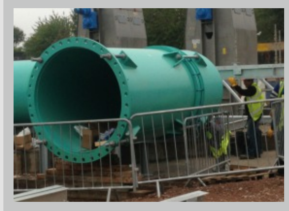
View of measurement place
