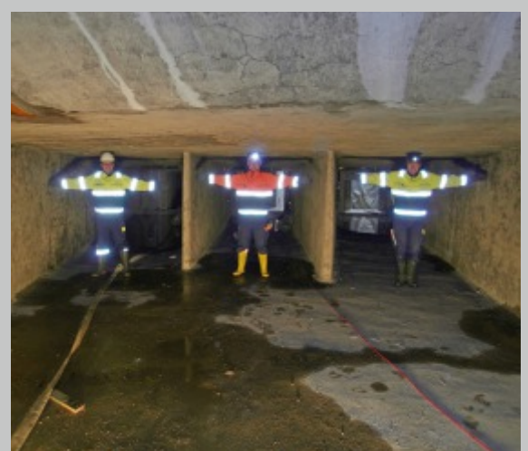
View of installation place
