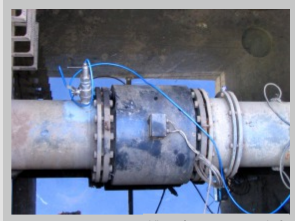
View of measurement shaft
