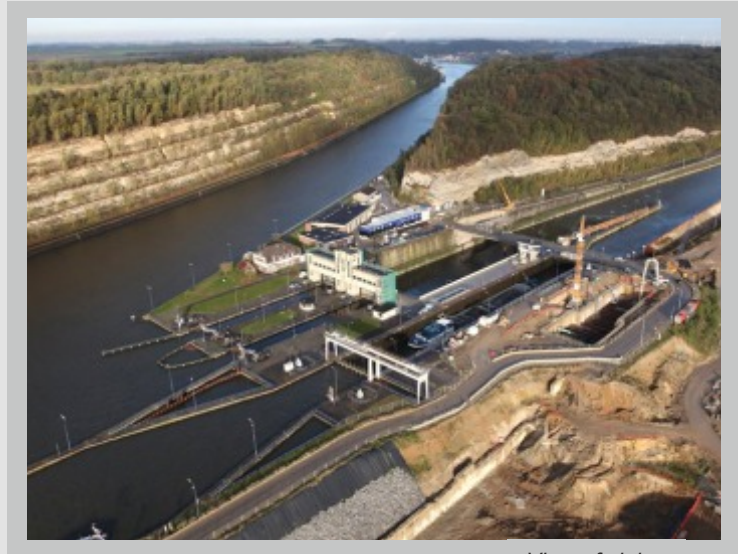
View of sluice
