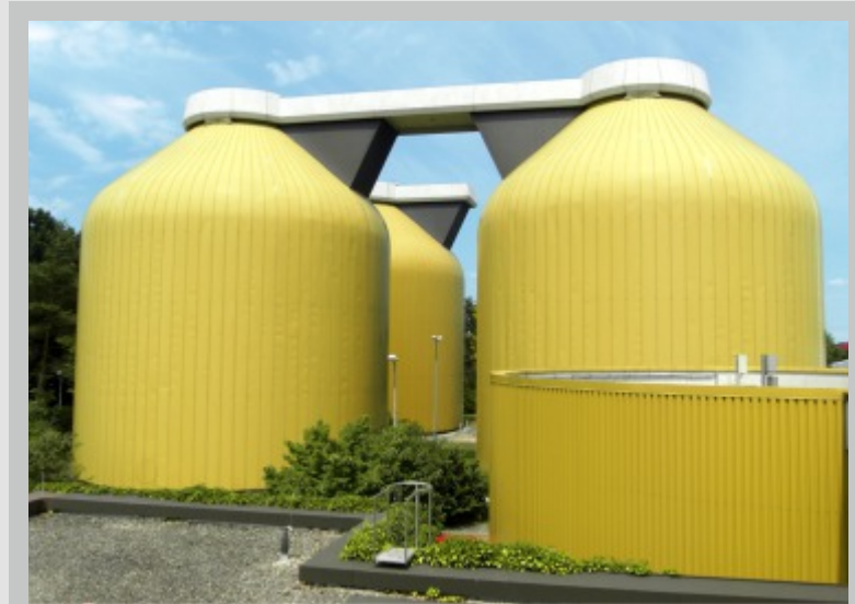
Pre-thickener in front of digestion tower (bottom right)
