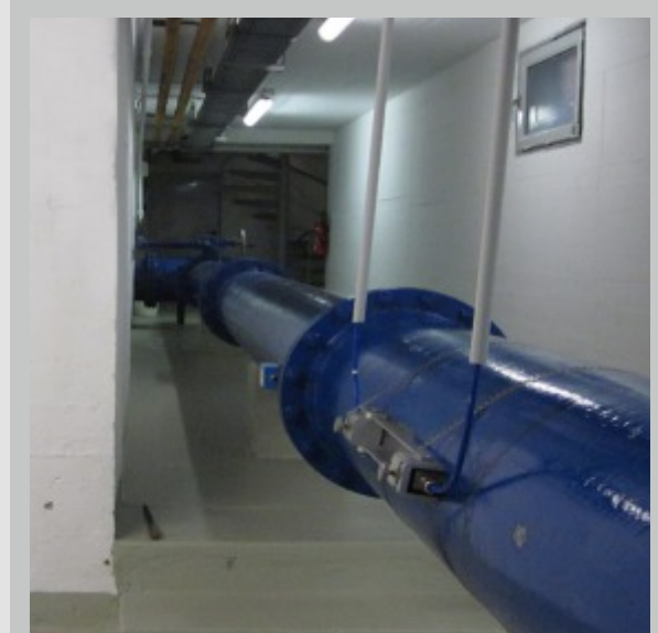
Flow Measurement using clamp-on sensors
