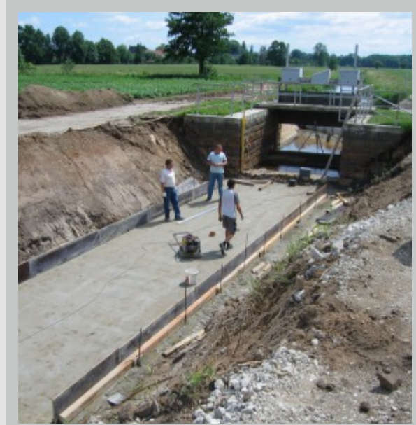
Measurement place under construction
