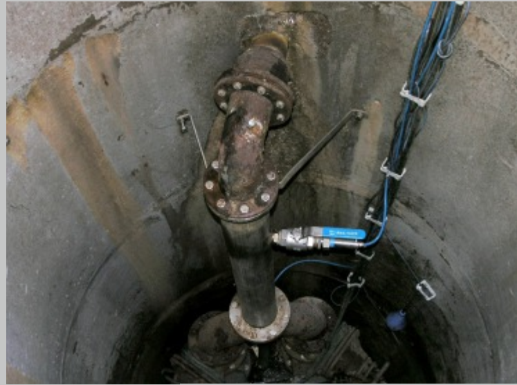
Pump shaft with built-in measurement system
