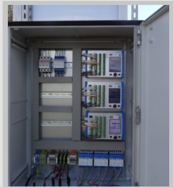
Transmitter installation in control cabinet
