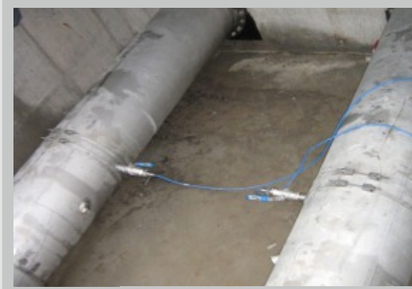
Measurement pit behind grit chamber
