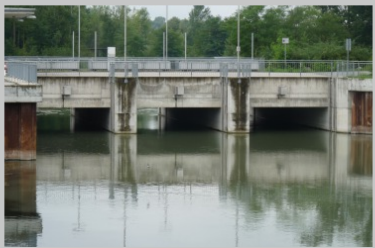
View of the 3 part flooded polder gates
