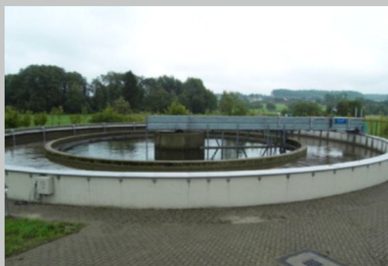
Two-chamber combi basin (activated sludge and secondary clarification)
