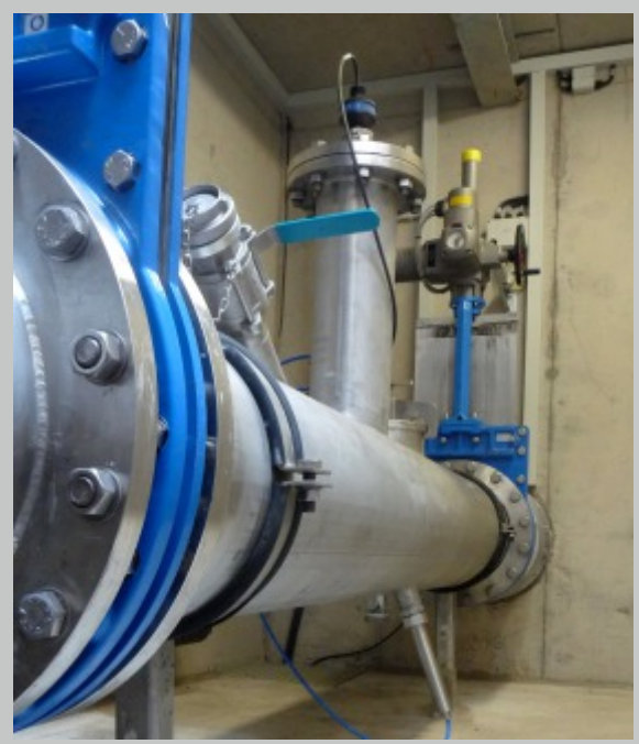
View of Measurement Place
