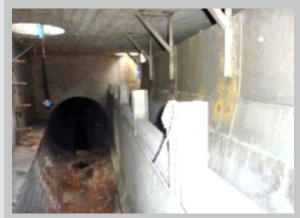
Stormwater overflow sill
