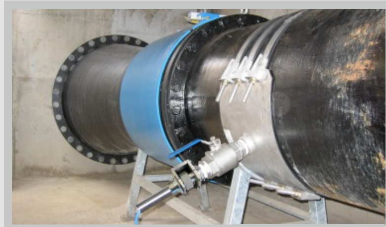
View of measurement place
