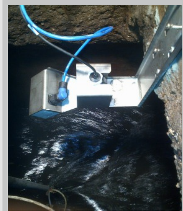
View into intake channel
