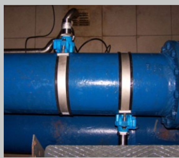
Filling and drain pipe with installed sensors
