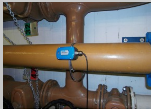
Installed Clamp-On System
