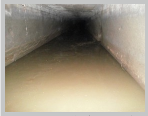
View of measurement place
